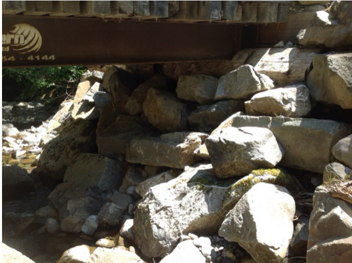
Right Bank Abutment when facing downstream
