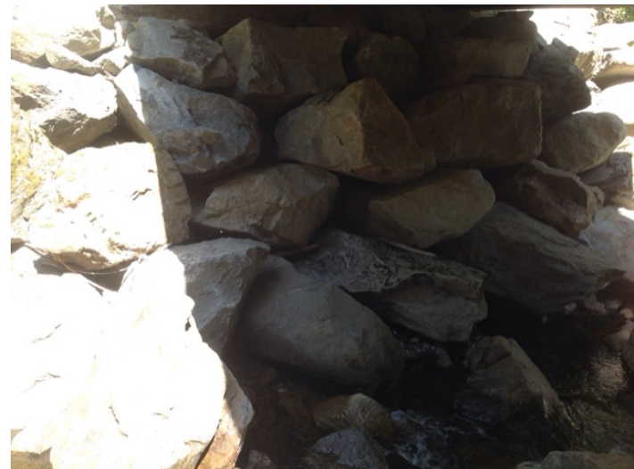
Left Bank Abutment when facing downstream
